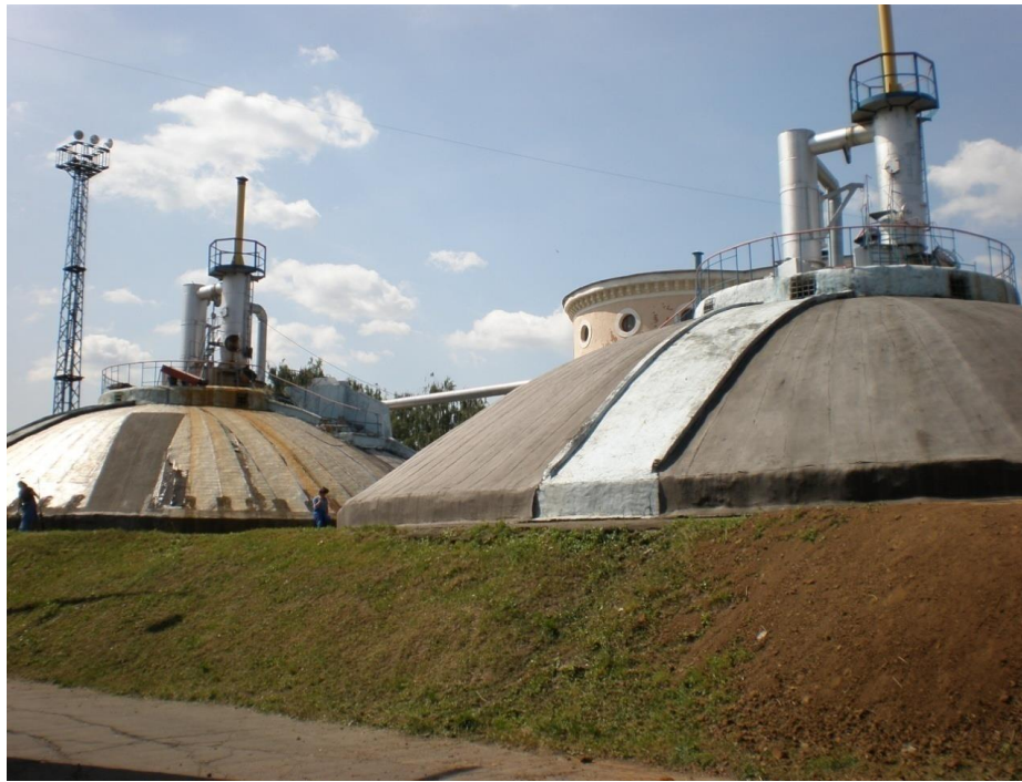
Fig. 3.13. Methane tanks in the form of reinforced concrete tanks buried in the ground.
