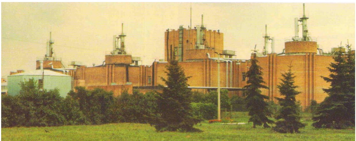
Fig. 3.14. Methane tanks in the form of above-ground tanks
